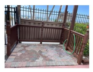
One of the first projects our new maintenance man, Jim Bennett, tackled was tearing out the old foot wash area by the beach and building a new one. The old area had composite boards on the bottom and had been warped and the railing around the area had deteriorated with the weather. Jim laid concrete pavers and built a new fence with railing to brighten up the area and help with drainage. THANK YOU!
