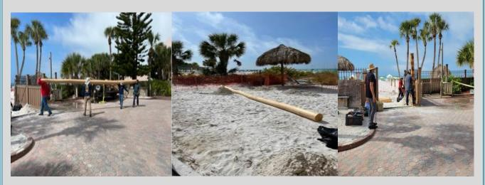
Precise measuring took place first and then each pole had to be hand carried to the work location. The first pole was inserted after drilling over 4 ft deep.
